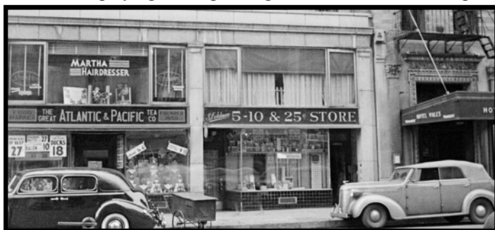
The original S. Feldman Housewares, 1929, located where Island restaurant now stands.
