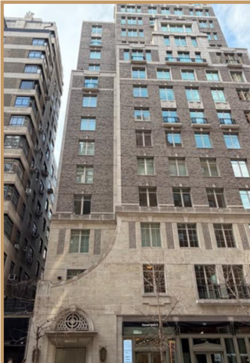
The front of 1228 Madison Avenue: the south window line left is set back 10 feet.
